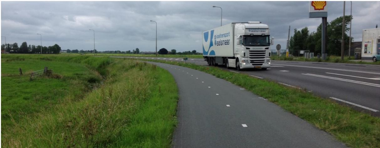
Typical inter-urban cycleway in the Netherlands. This is a “cycleway that can be used by pedestrians”. It provides meaningful protection from higher speed vehicles including HGVs, given greater emphasis and safety by the grass strip between cycleway and road. The garage opposite has its own cycleway access, recognising that cyclists may also want to use the shop.
