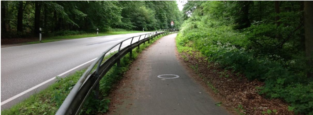
Denmark: Cycleway that can be used by pedestrians. This example has gradients, curves and underpasses designed for easy cycling, but it can also be used by equestrians, wheelchair users and other pedestrians who are few in number. The guard-railing provides a safety buffer against high speed traffic where land ownership forces the path to be close to the carriageway.
