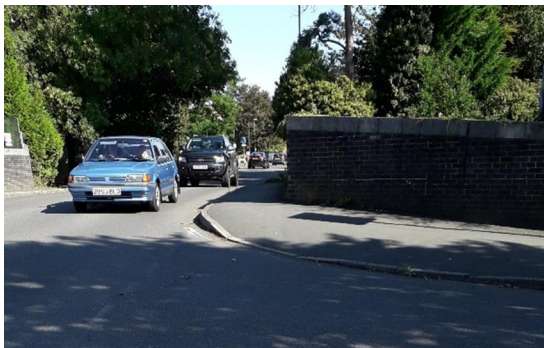
Wimblehurst Road rail overbridge
