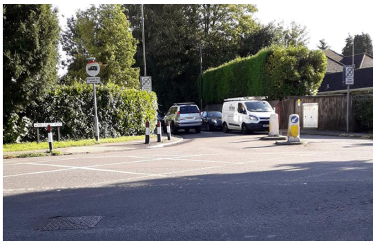
Wimblehurst Road arm of North Parade signal junction - no signal crossing and narrow pedestrian refuge
