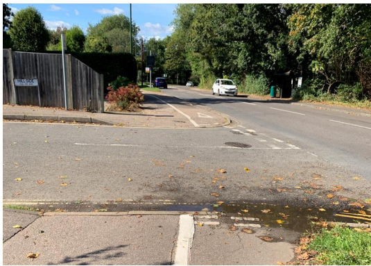
Existing narrow segregated path on Guildford Road, without priority across side roads
