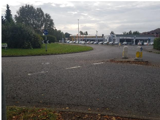
Parsonage Road roundabout - long pedestrian crossing distances
