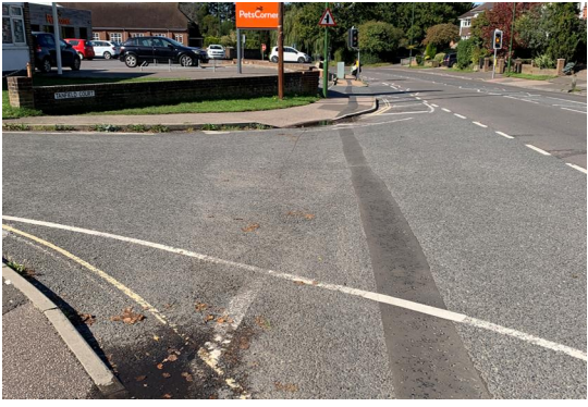
Wide side road crossing at Tanfield Court
