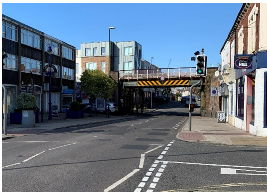
Queen Street railway underbridge (The Iron Bridge)
